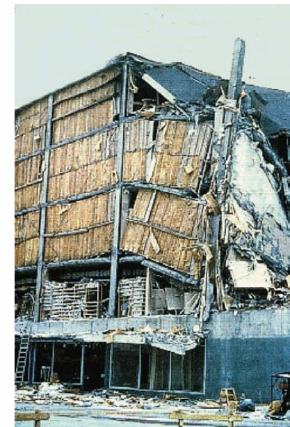
Figure 5-18: Penney's store, Anchorage, Alaska, earthquake, 1964. Left: Damage to the store: loss of perimeter precast panels caused two deaths. Right: Second-floor plan, showing unbalanced perimeter resistance. SOURCE: JAMES L. STRATTA
